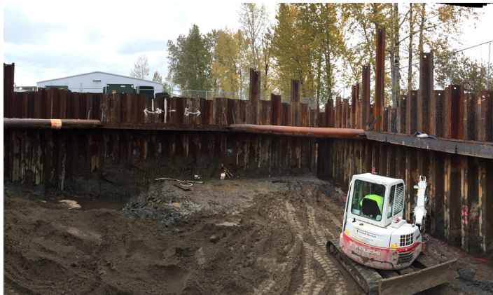
Remediation activities at aluminum extruding and anodizing facility.
